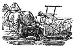
ga Chief, (an excellent Cayuga Chief-Combined Mower and Reaper. two-wheeled machine) as a reaper, in which the operation of hand-raking is distinctly represented.
